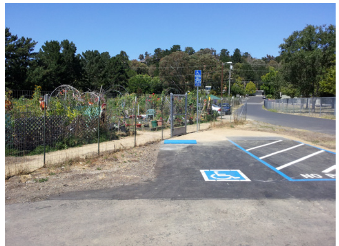
New van accessible parking space next to new gate and new decomposed granite path.
