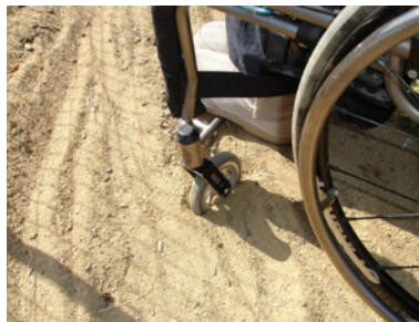
Wheelchair wheels sinking into the old path material, loose dirt.
